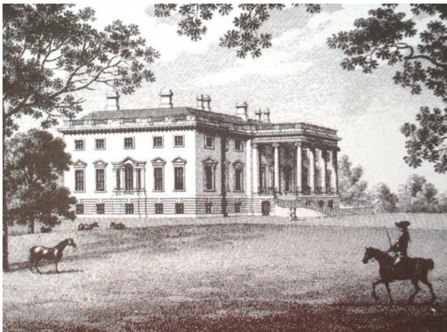
Wricklemarsh: Some of the columns and windows came to Beckenham Place the large ground floor window is the same as at the sides of portico
