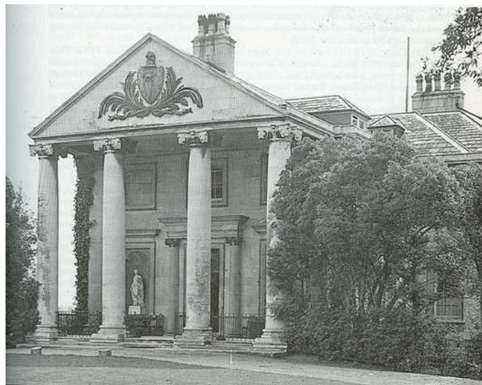
Beckenham Place circa 1892 – if accurately dated this photo shows the roof dormers installed prior to the house being used as a school or sanatorium.
