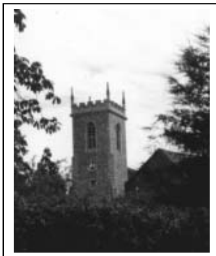
The newly installed church clock
