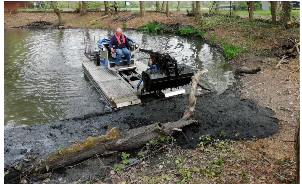
Clearing the silt from the pond
