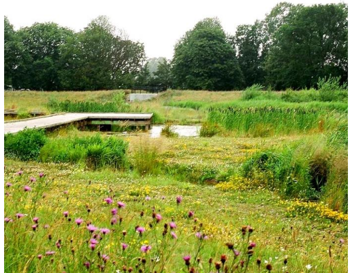
Recreated wetland within part of the flood storage area at Sutcliffe Park, Kidbrooke. The park's 2.5m (8ft) high flood embankment can be seen in front of the trees.
