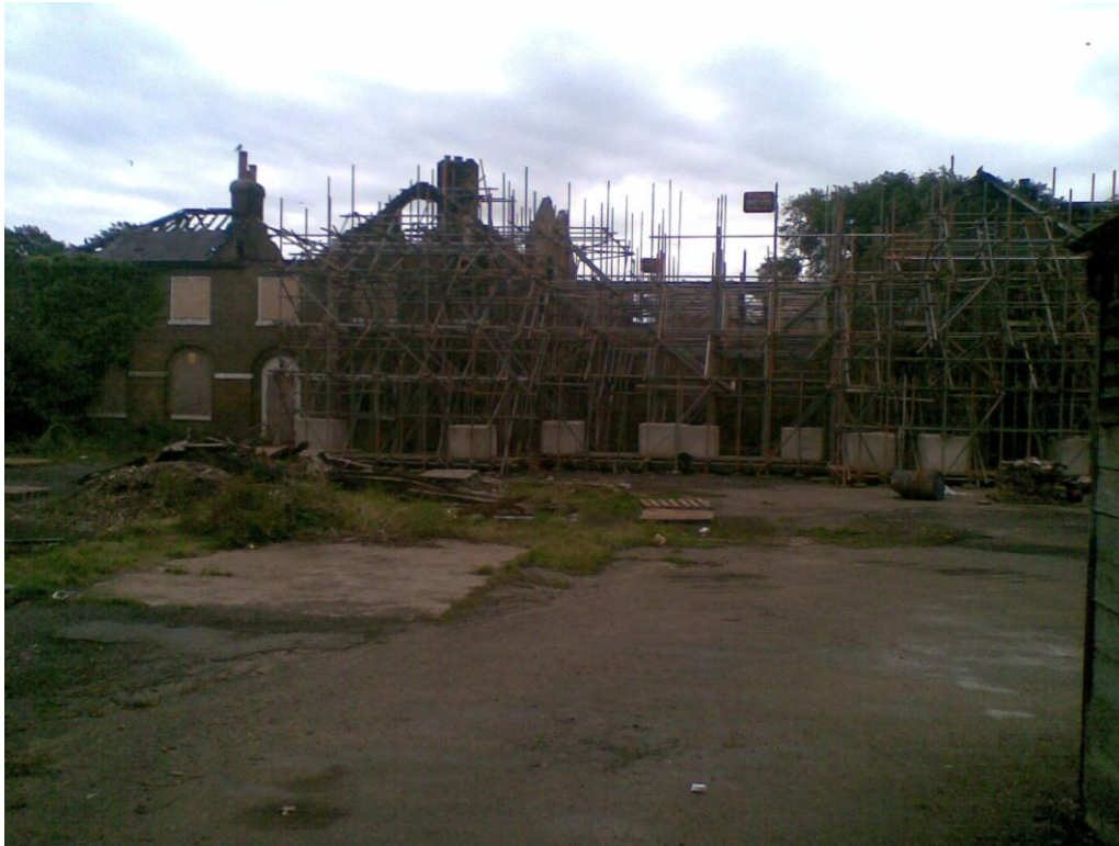
After the fire, supported by scaffolding
