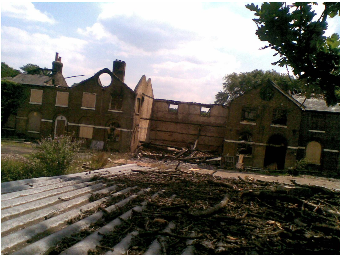
The day after the fire
